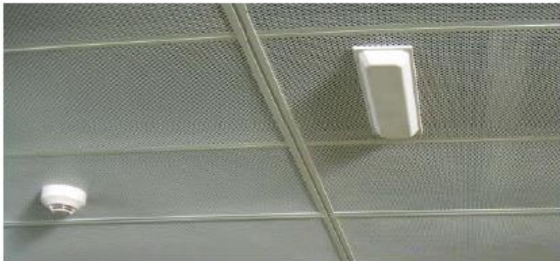
Figure 12 AP-ANT-16 Downtilt Antenna Flush-Mounted to Ceiling Grid
