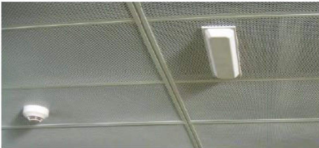
Figure 12 AP-ANT-16 Downtilt Antenna Flush-Mounted to Ceiling Grid
